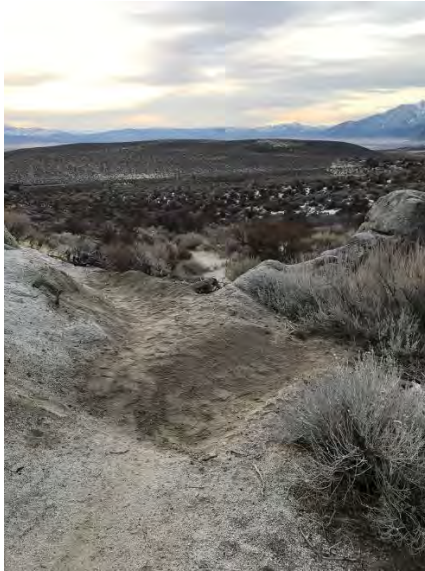
Trail widening, drainage work and armoring
