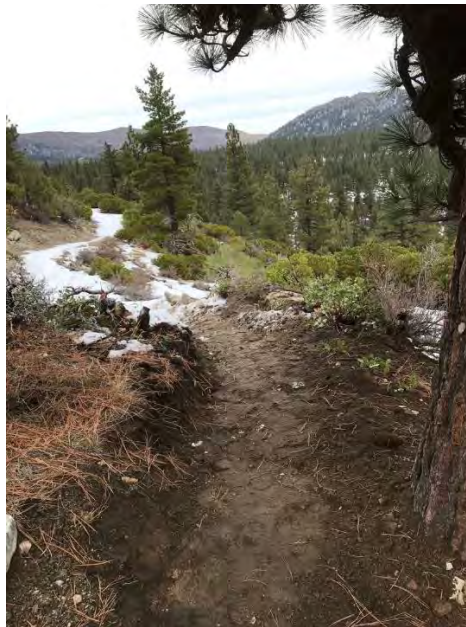
Trail widening and safer sightline
