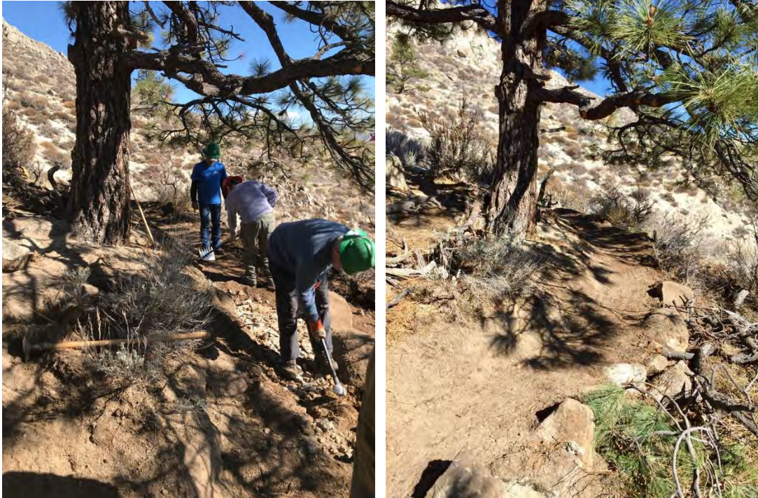
Trail realigned below tree
