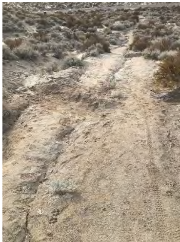
New drains on old road...
