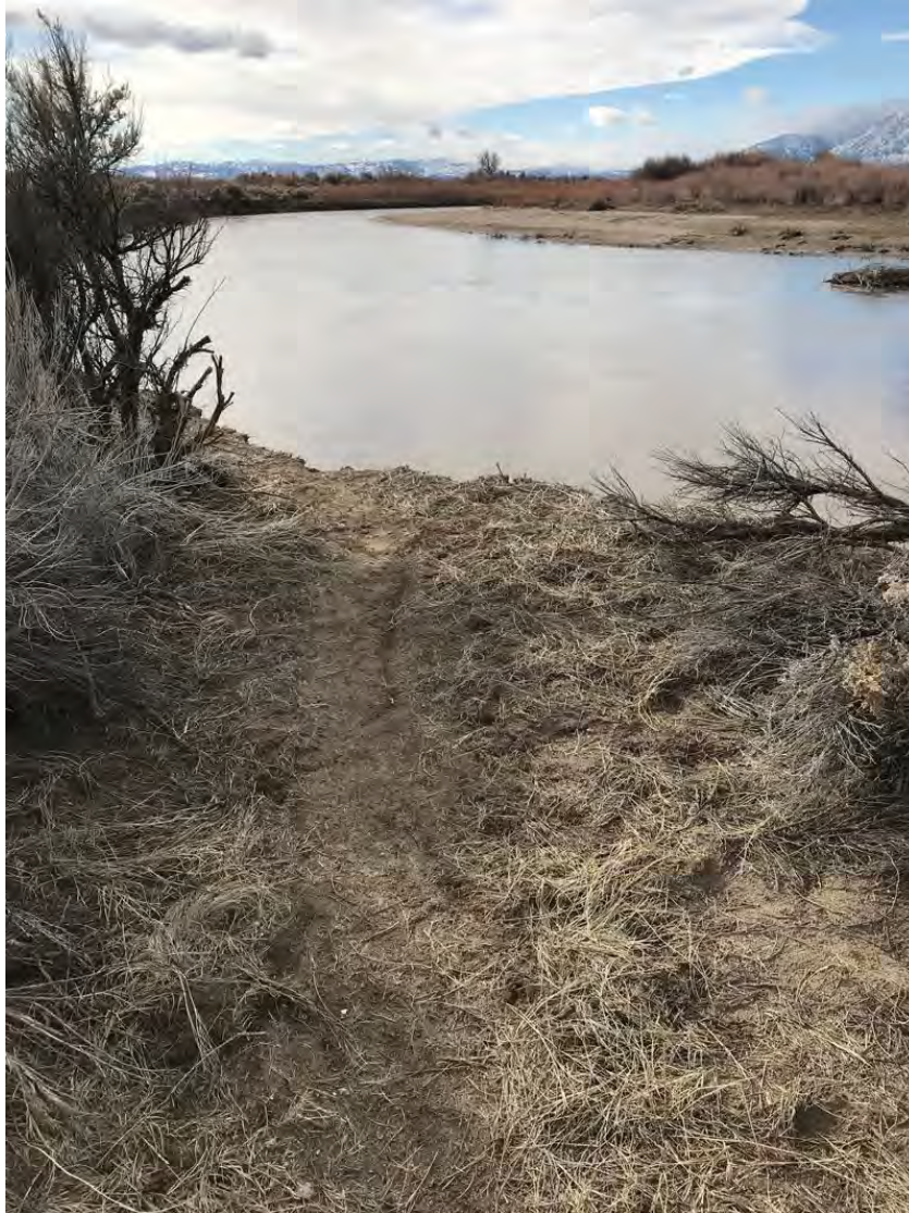
Section of trail washed away and rebuilt
