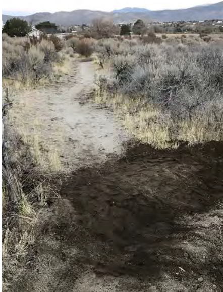
Trail drainage maintenance
