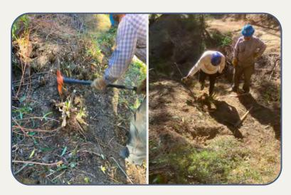
Sections of slickrock were chiseled out on the Appaloosa Trail to improve and widen the trail tread. The first 1.5 miles of trail above Jobs Peak Ranch Trailhead was brushed out and any rockbergs removed.
