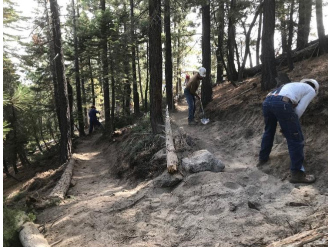
Realignment of a switchback
