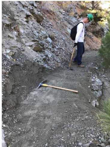
Benching work through rock slide area
