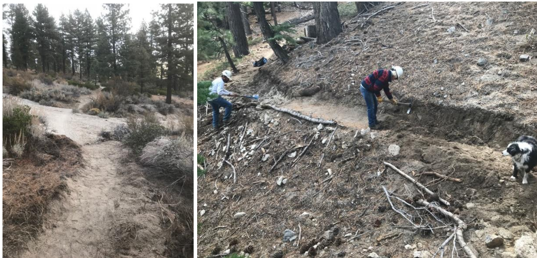
Benching and widening trail
