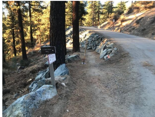
Trail armoring at road crossing
