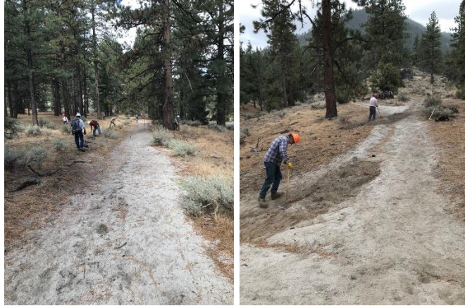
Social trail decommissioning and drainage work
