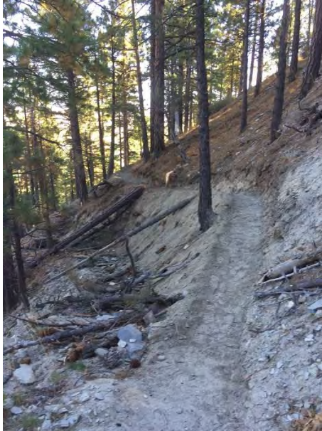
Landslide Area Realigned
