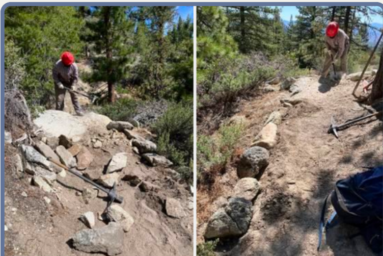
Tread widening and rock removal
