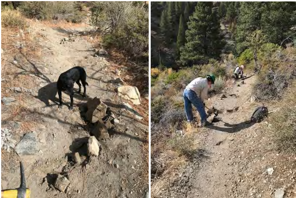
Rock obstacles removed from trail
