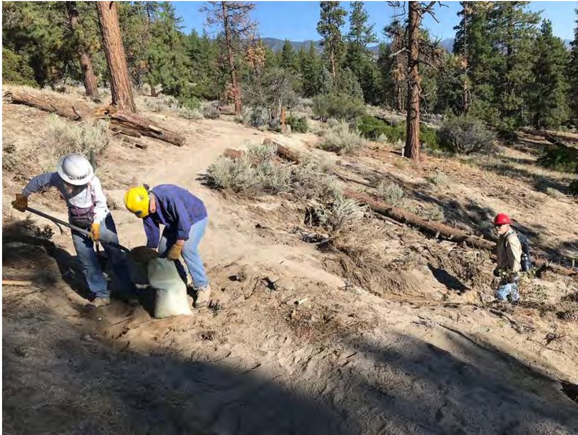
Refilling mudslide gash across trail
