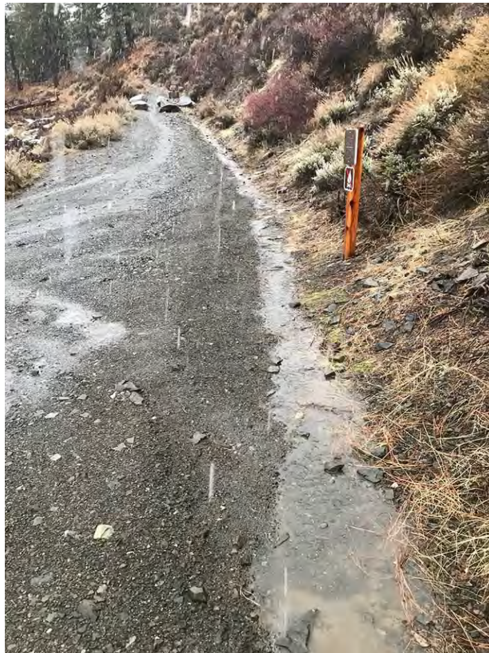
Brush removed for unimpeded water drainage
