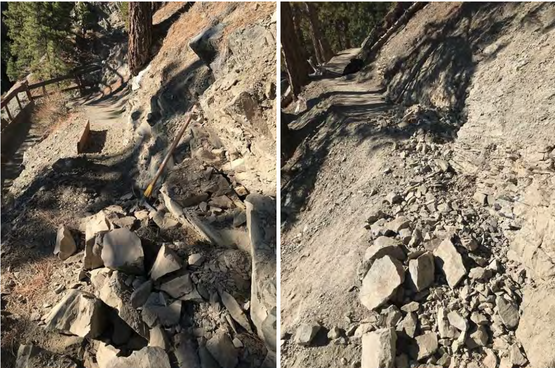
Sections of trail chiseled out and widened
