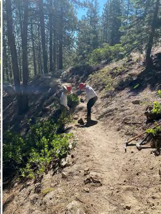
Widened and armored section
