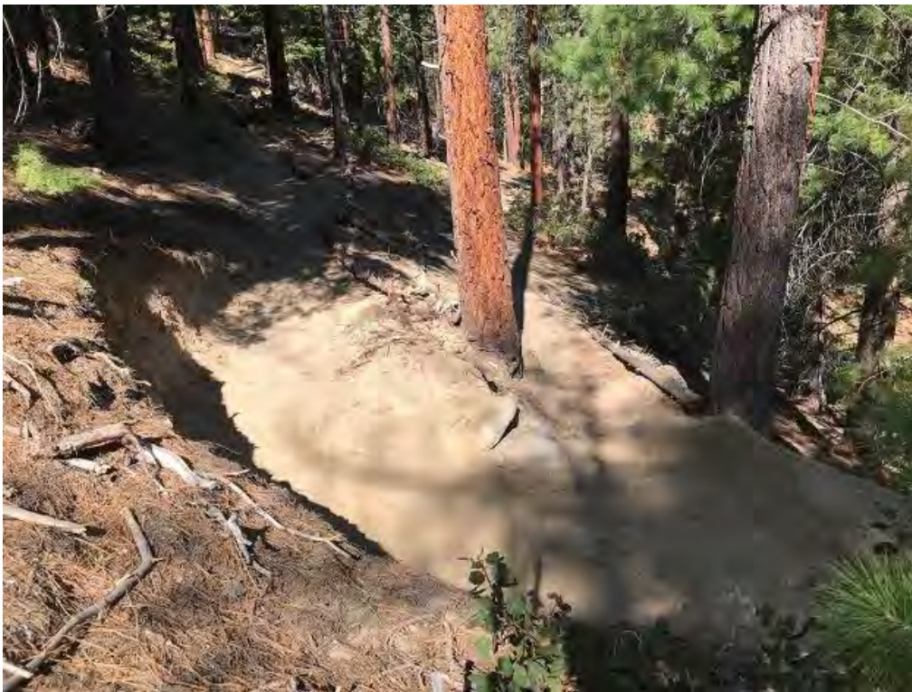
Switchback widened and armored
