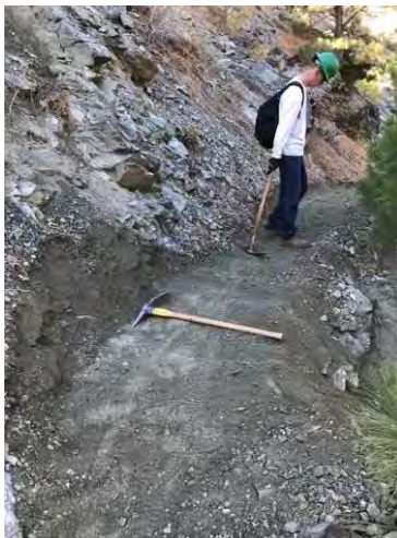
Benching work through rock slide area
