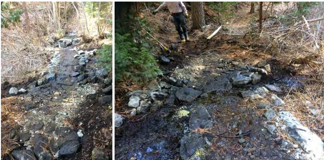
Rock causeway expanded
