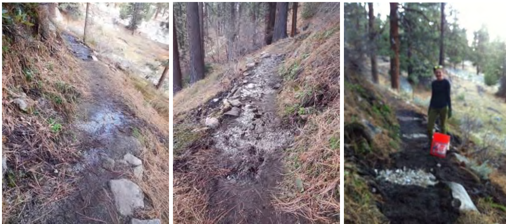
Bogy trail section filled with crushed rock
