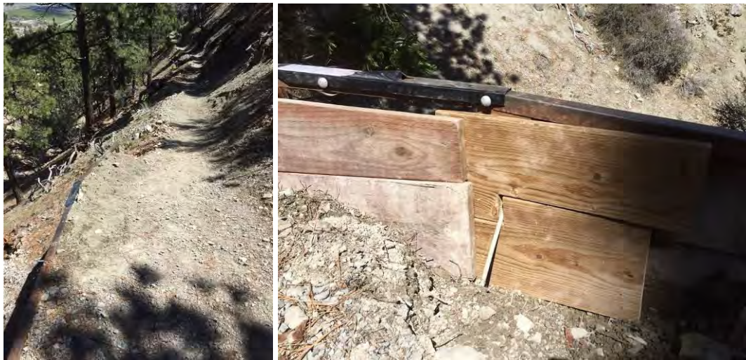
Retaining wall repaired
