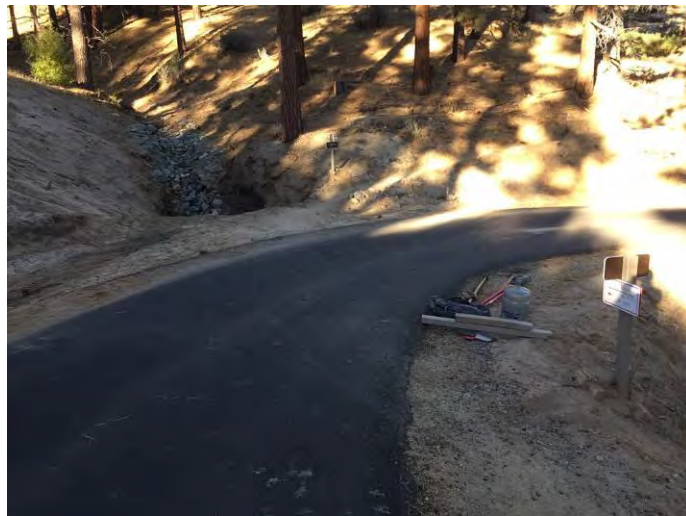
Trail realigned below new catch basin
