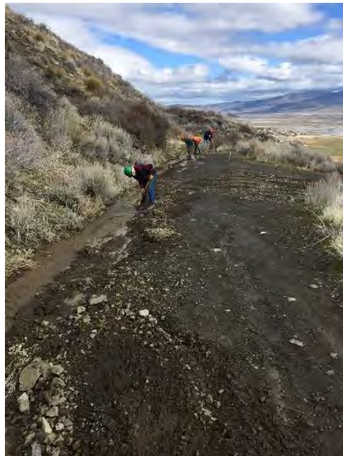
Before and after: A berm was built to contain water and prevent further damage to an old road section of trail directly above Eagle Ridge TH.
