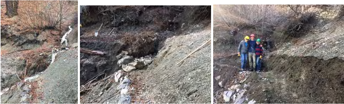
Before, during and after: The third crossing above Eagle Ridge TH was severely damaged from flooding. The crossing was armored and trail repaired
