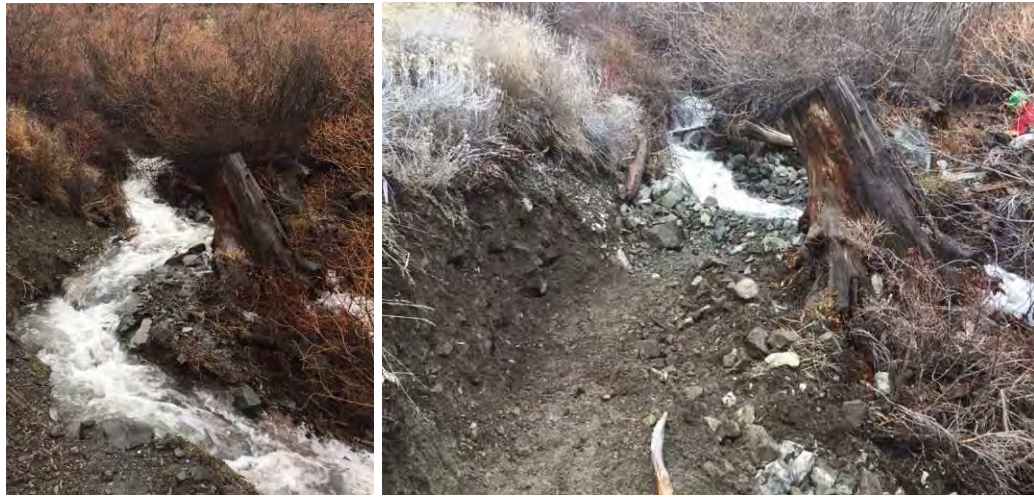
Before and after: The Adams Canyon crossing overflowed onto the trail. The water was redirected into its channel and the trail repaired
