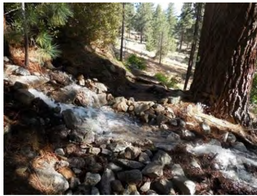
Rocks placed to prevent water on the trail
