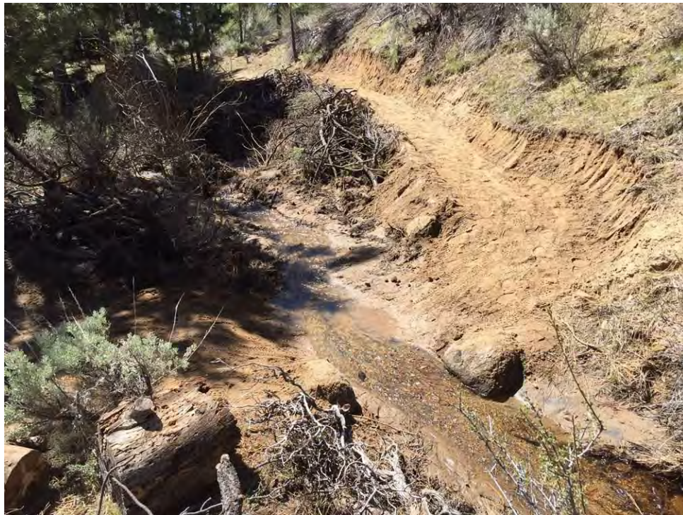
Trail benched back, debris cleared and rock crossing installed
