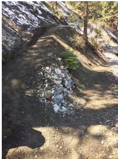
Grade reduced on second switchback
