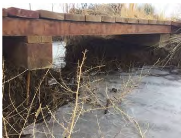
Damaged boardwalk footings
