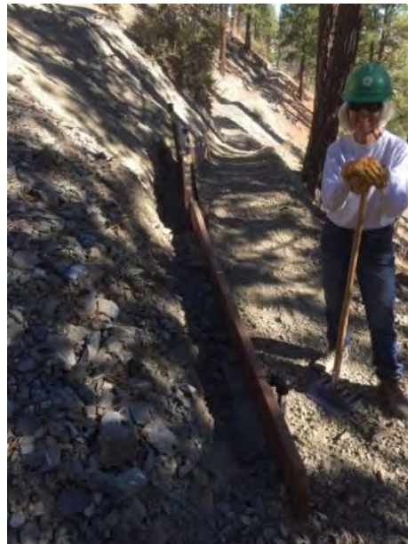
Rebuilt support wall
