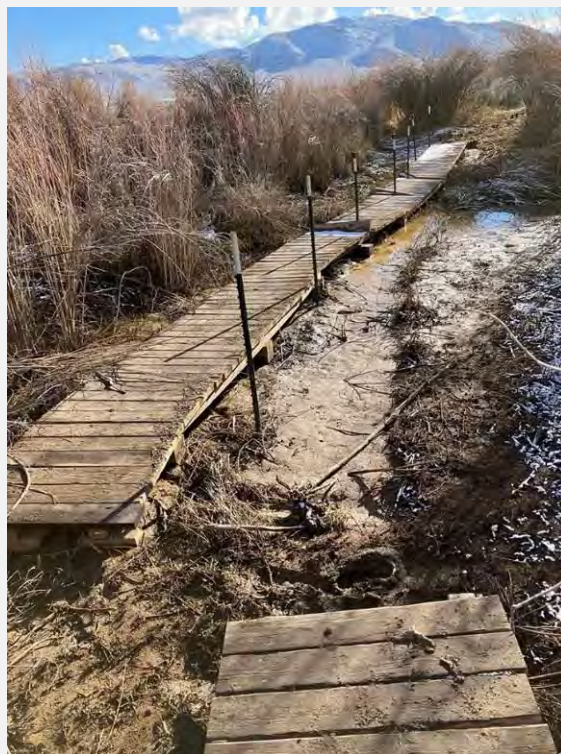
Boardwalk damage
